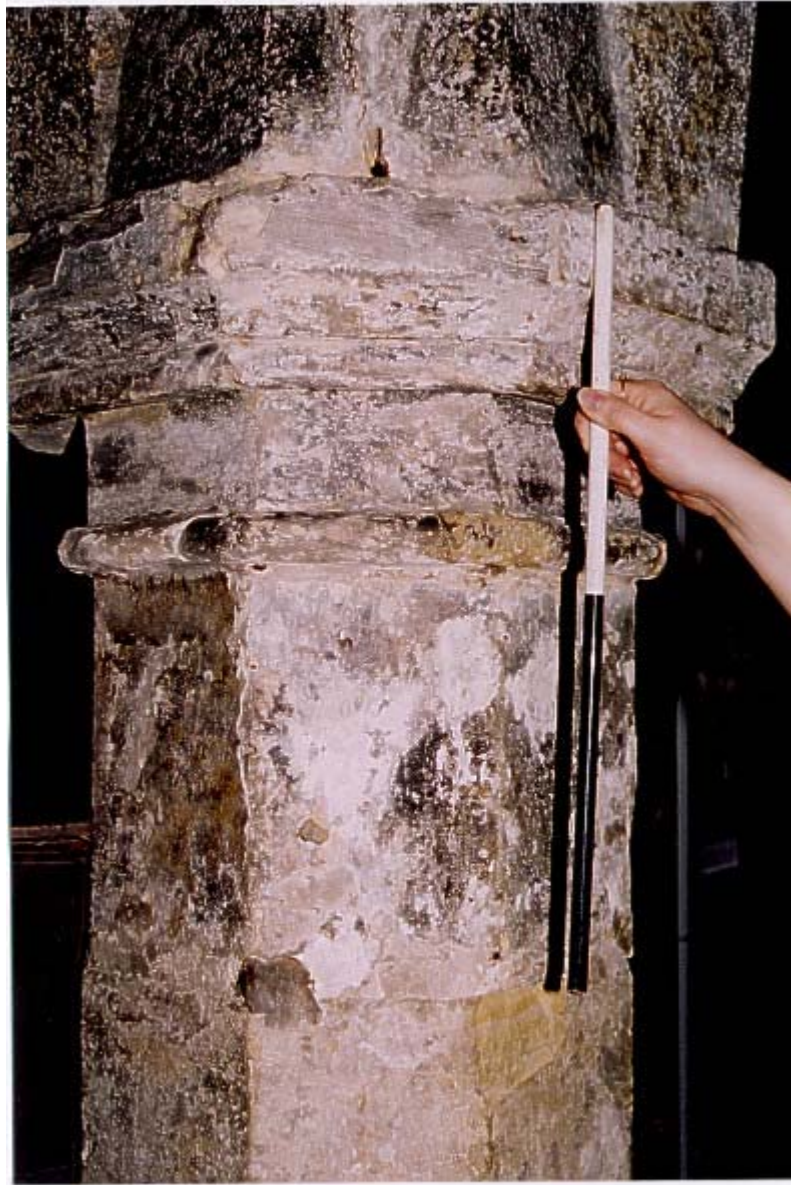
Fig. 15: Pier 7, detail of south face
