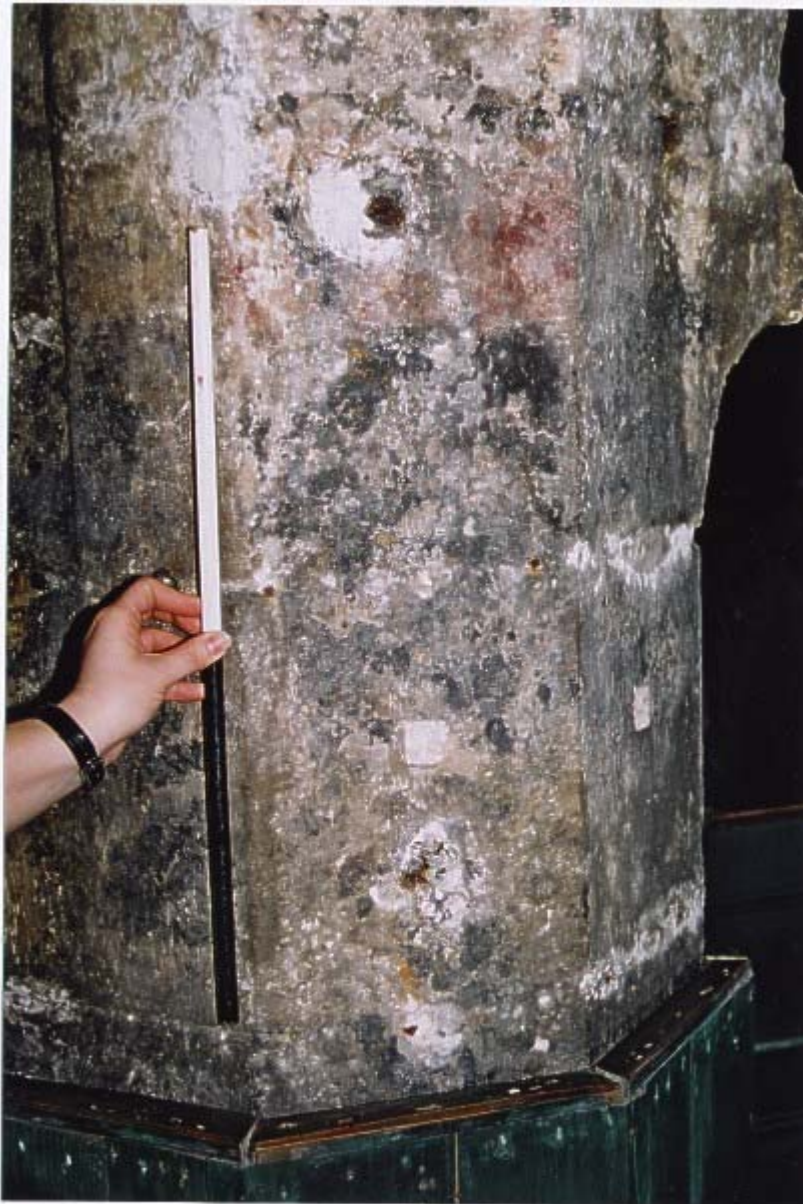
Fig. 6: Pier 2, detail of west face
