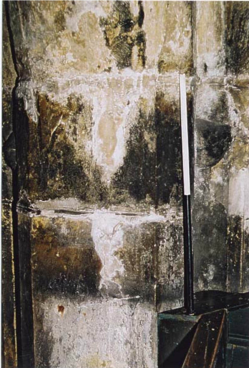
Fig. 5: Pier 1, detail of east face
