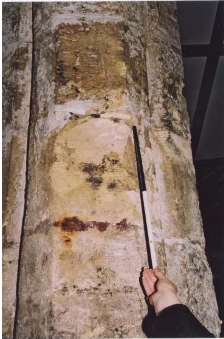
Fig. 11: Pier 2, detail of east face
