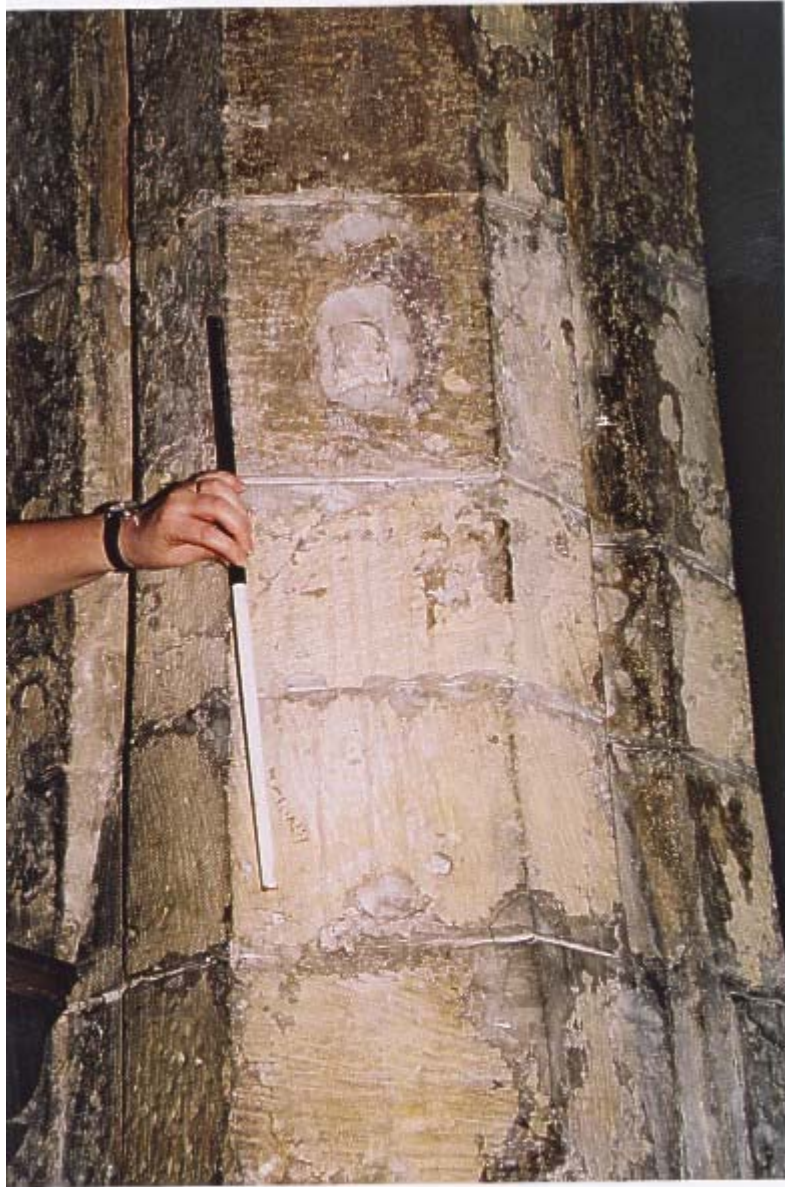
Fig. 12: Pier 3, detail of west face
