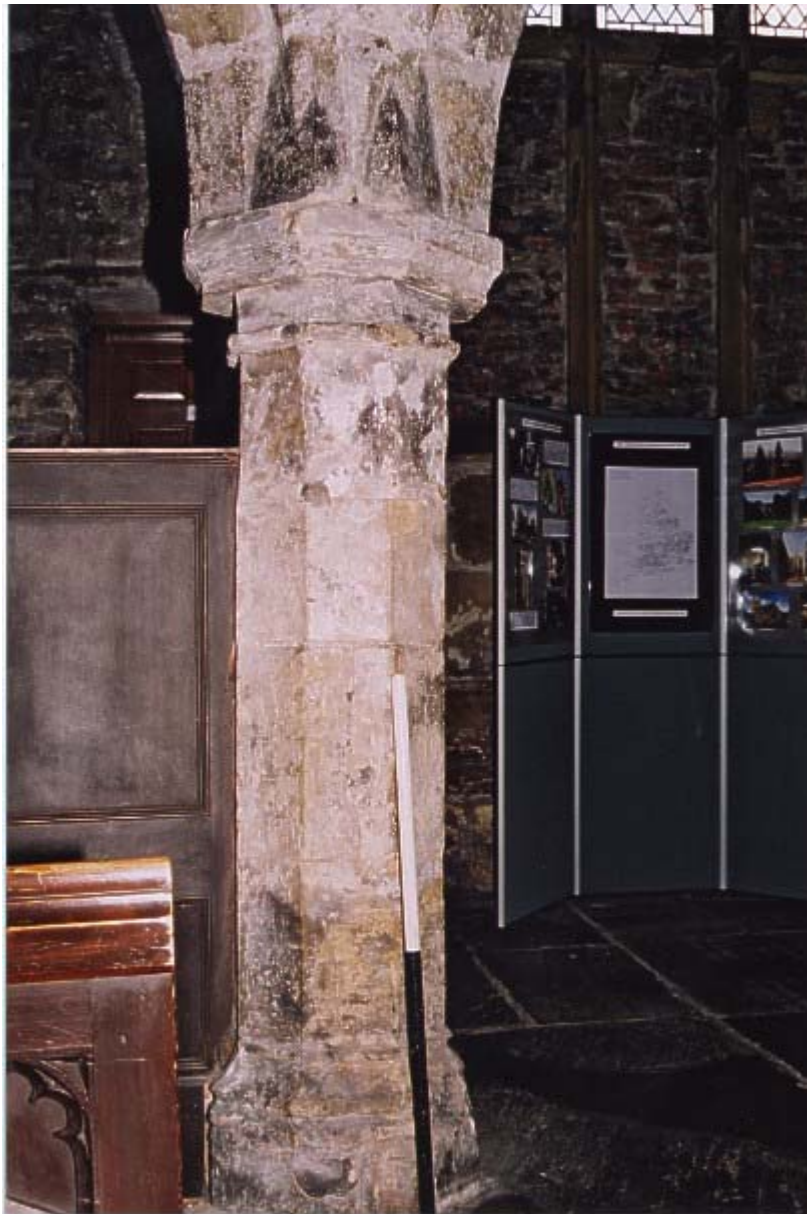
Fig. 14: Pier 7, south face
