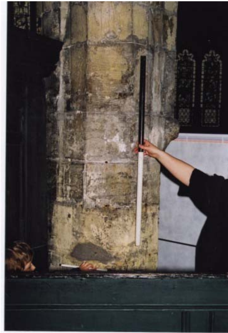
Fig. 10: Pier 3, west face
