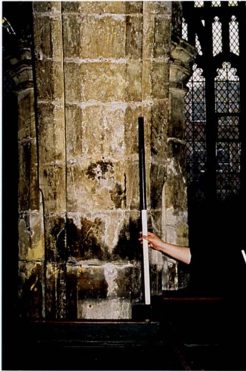
Fig. 4: Pier 1, east face
