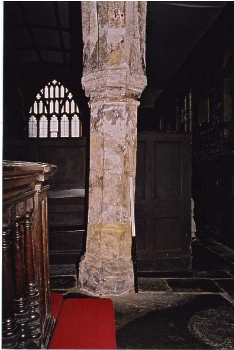
Fig. 13: Pier 7, east face
