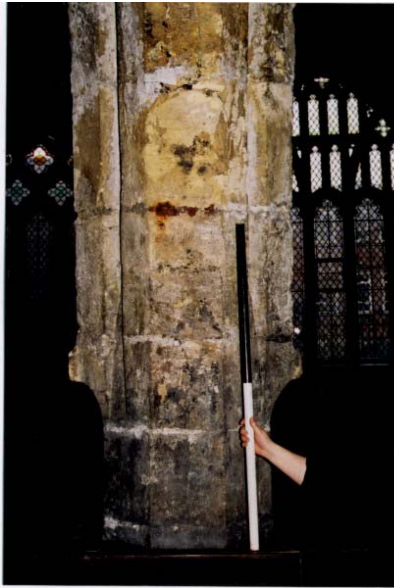
Fig. 9: Pier 2, east face
