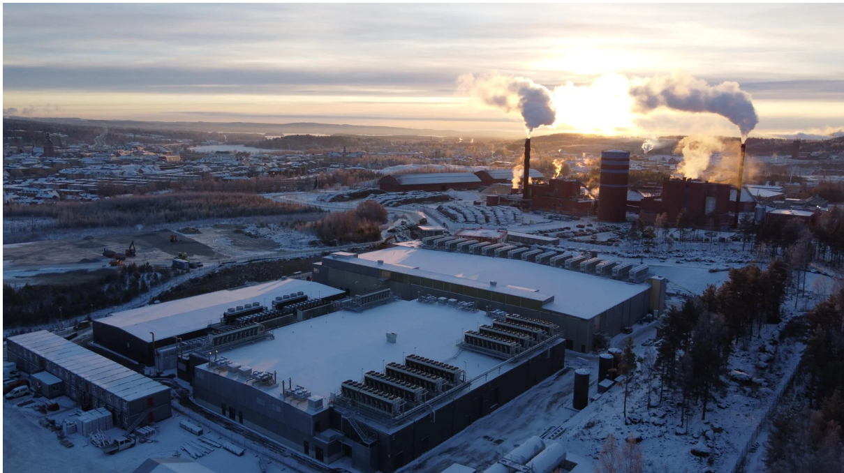
Figure 1. EcoDataCenter in Falun Sweden. The Datacenter where Viking 2 is located sits in the foreground of the image. The sawdust mill is located in the back of the image. Heat produced by Viking 2 is piped into the sawdust mill to dry wood and create pellets for renewable energy generation.
