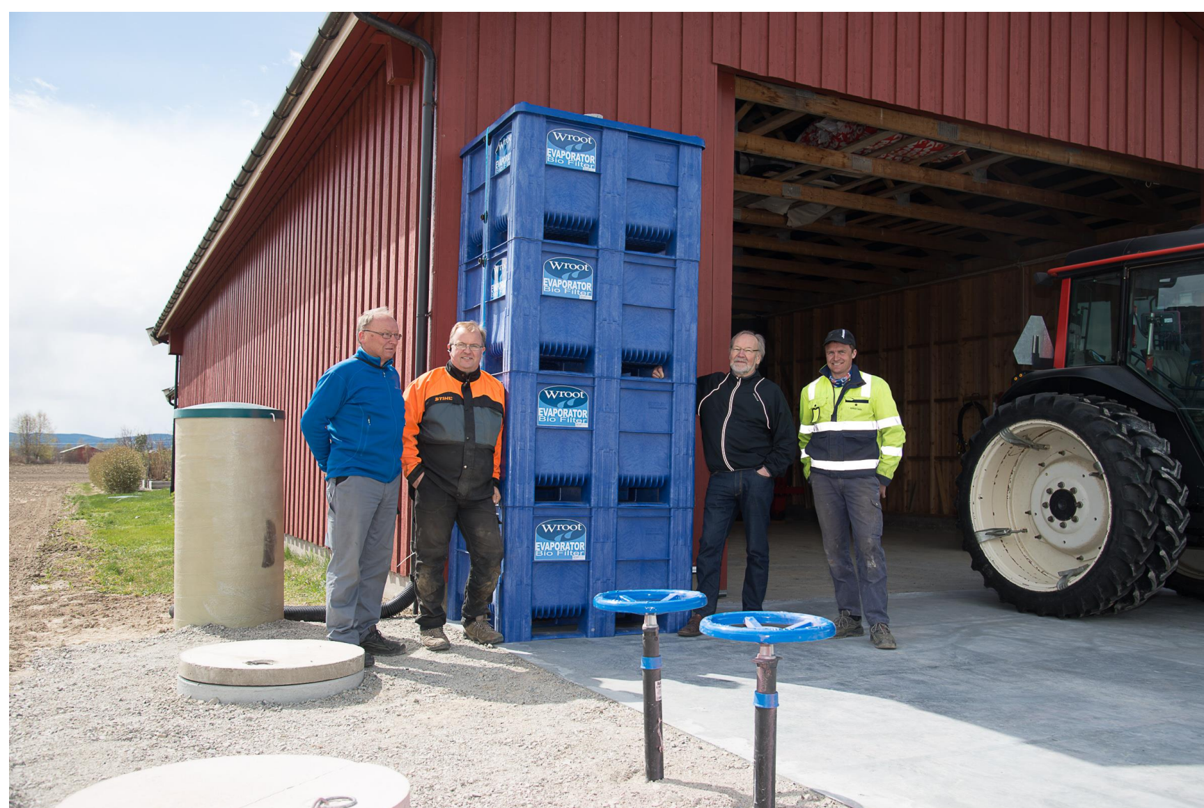
Figure 3. Containers filled with biomix and stacked to allow gravity flow and recirculation (Photo E. Fløistad).
