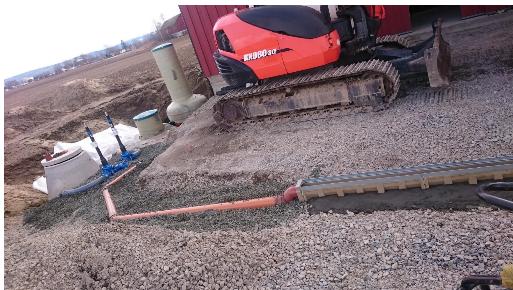
Figure 2. Construction of the sprayer fill area with drainage to the silt trap and liquid container (Photo K. Sveen).
