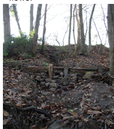
Fence in a wooded buffer to stop gully and to disperse the flow
