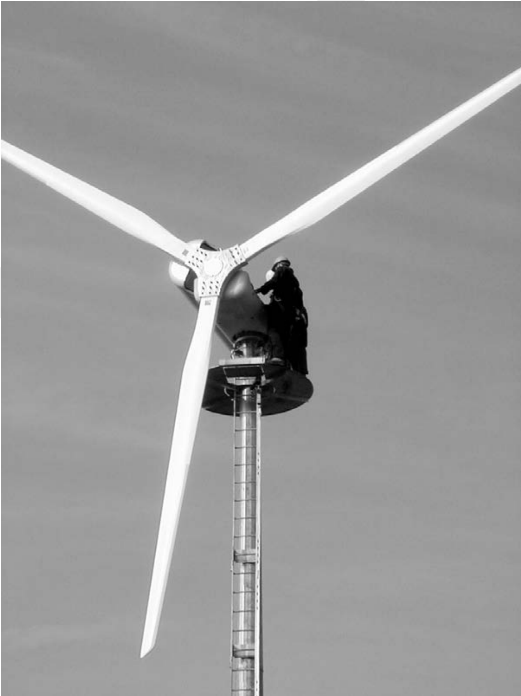
Fig 2: Maintenance of a wind turbine in progress
