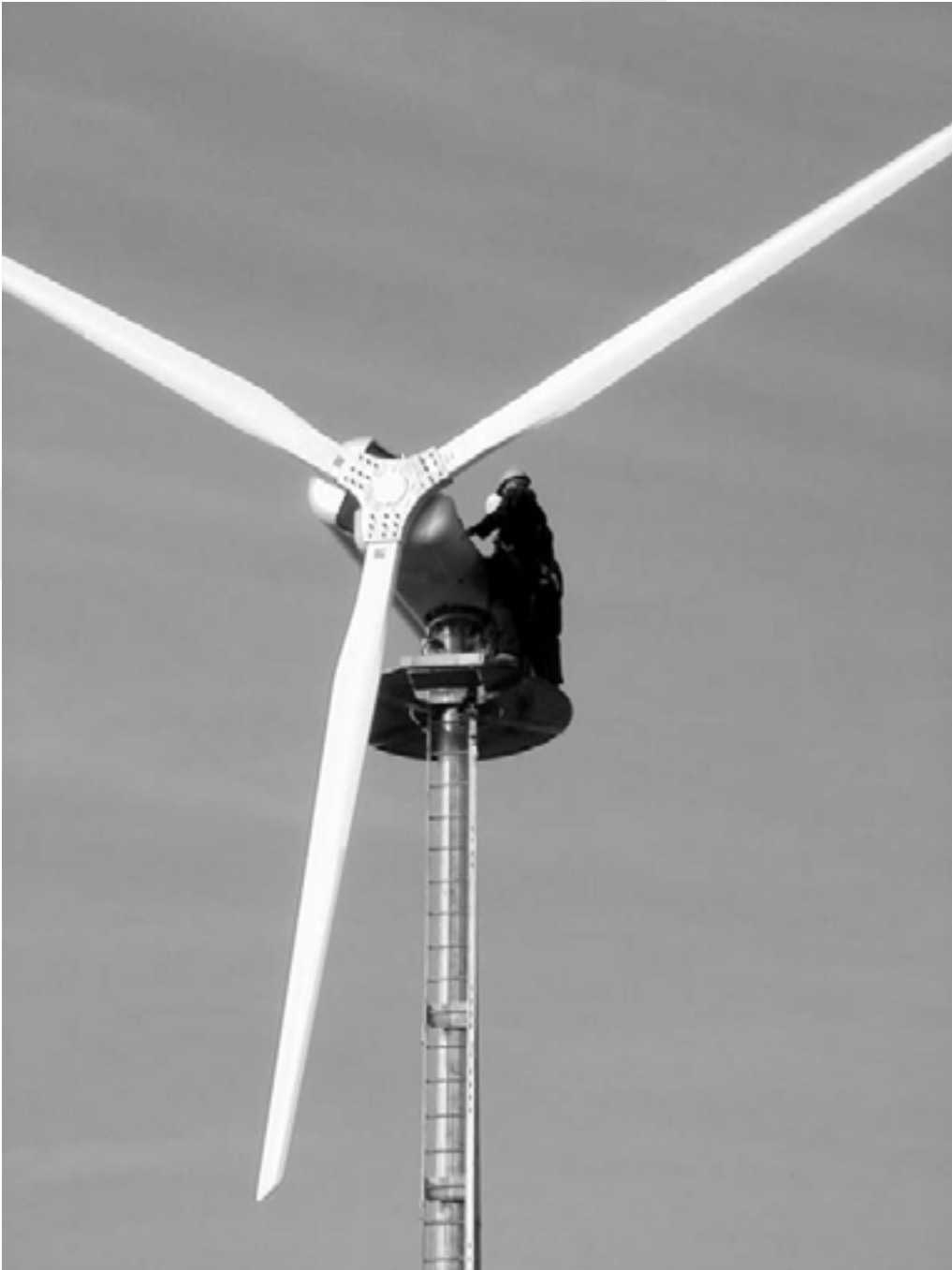
Fig 2: Maintenance of a wind turbine in progress
