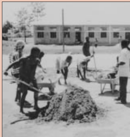
Rural development – building a new school in Burundi.
