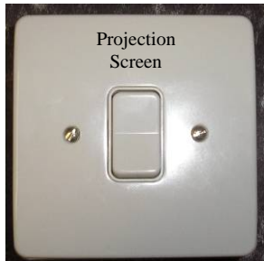
Figure 2- Typical Projection Screen Switch
