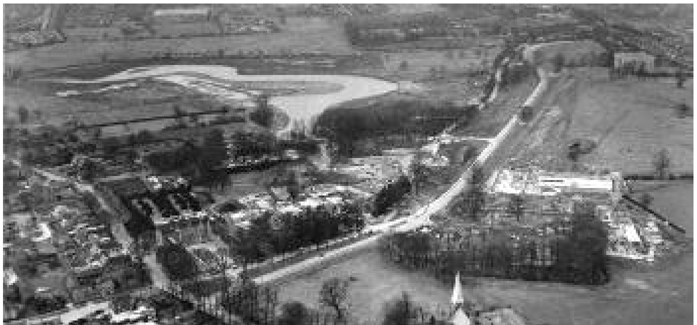
↓ Campus West during construction in the 1960s
