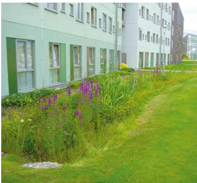
↑ Figure 18 Swale outside Goodricke College in phase 1 development
