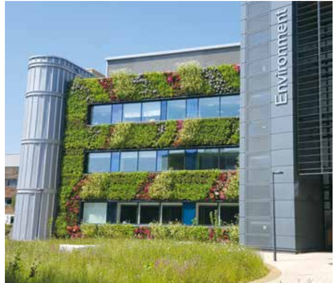
↑ Figure 30 The Living Wall on the new Environment Building
